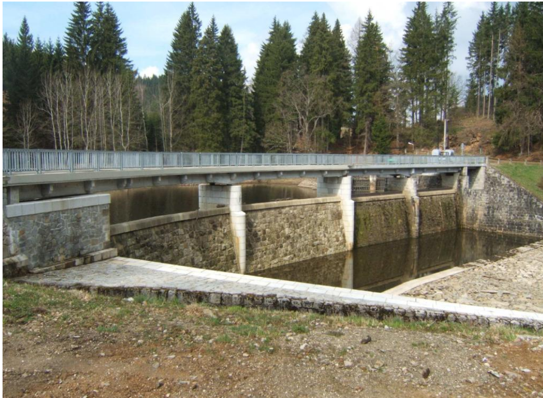
Picture 4 – Soběnov – new concrete hydraulic structure after the collapse during 2002 flood – Jiří Švancara
