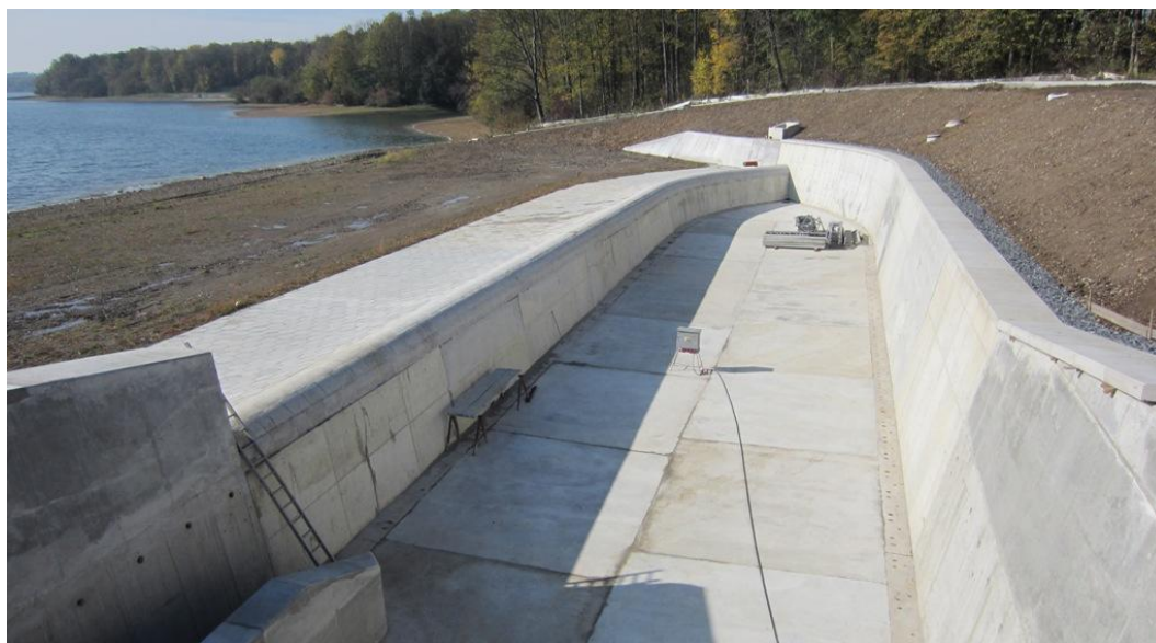
Picture 7 – Těrlíčko – rehabilitation of the emergency spillway designed on results of the scale model – under construction
