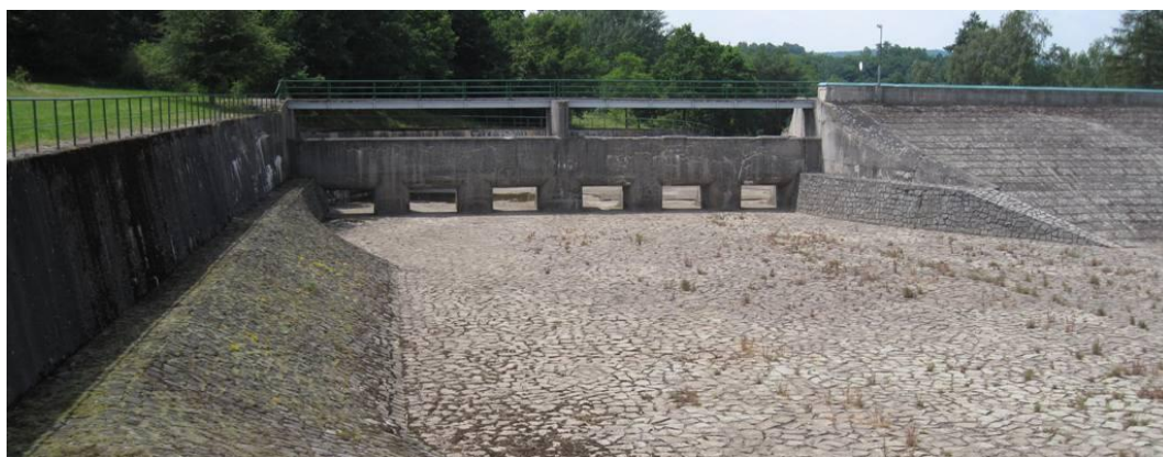
Picture 5 – Klabava – emergency spillway – before reconstruction
