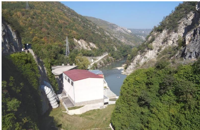
Figure 2. The new penstocks and power plant of Matka dam; behind is the old power plant, now a museum (view from the dam crest).
