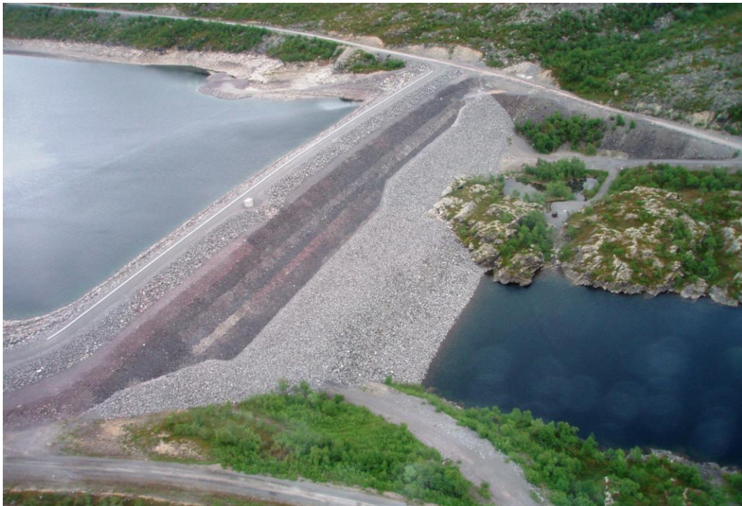
Picture 1 One of the Suorva rockfill dam in northern Sweden exemplifies a Swedish hydropower dam
