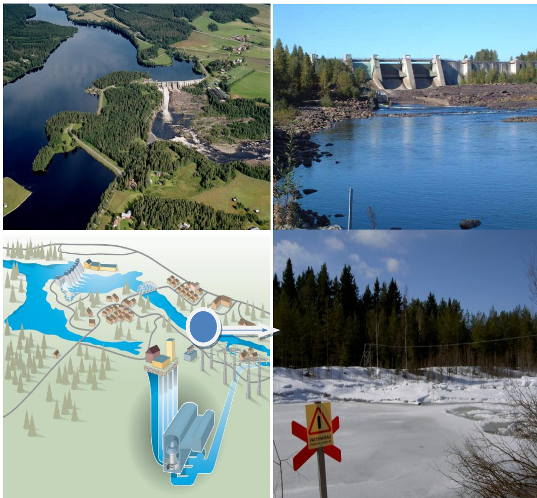
Picture 5 Pictures showing the area of the Stornorrfors dam and the dam and spillway from downstream.
