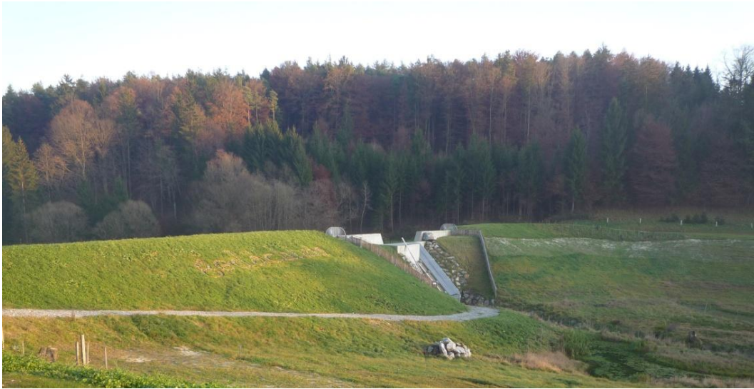
Picture 6 Retention basin Labuchbach
