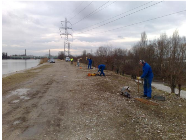
Picture 2.1.1 Installation of an array of temperature probes
