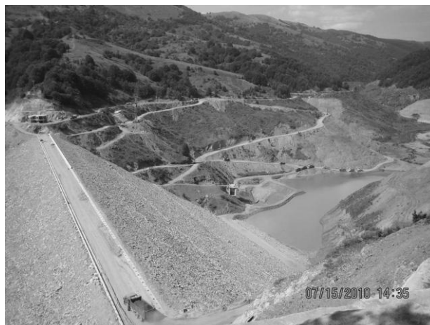
Picture 3.2.1 Knezevo Dam during construction (July 2010)
